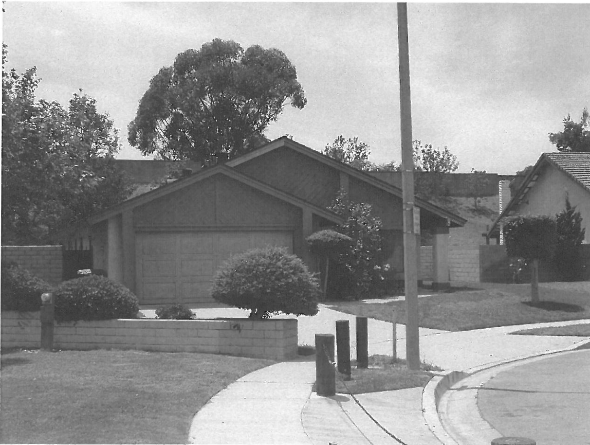
1 View facing southwest of side yard and front of residence
